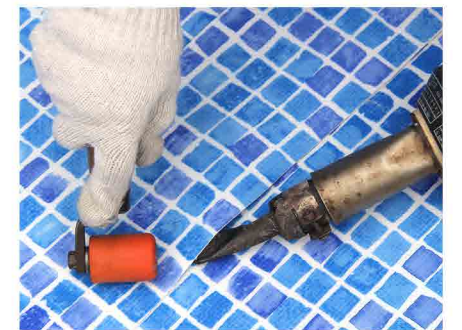
6. 池底铺设焊接 Floor laying and welding
