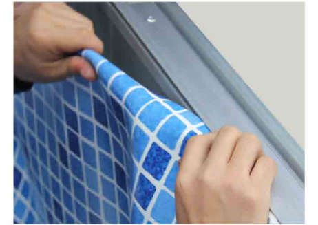
3. 胶膜固定件安装 Installation of hung profile or PVC coated metal
