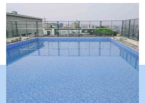
9. 试水验收 Acceptance inspection
