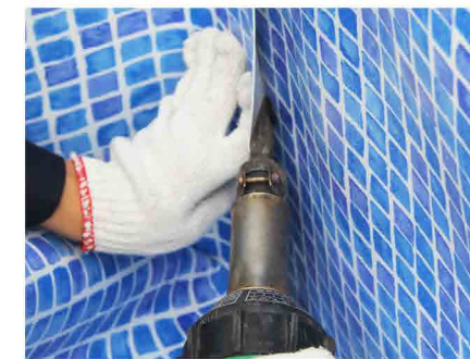
5. 池壁铺设焊接 Wall laying and welding
