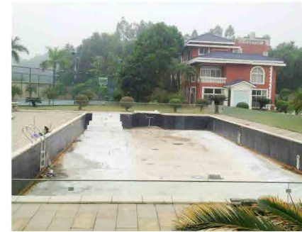
1. 基面平整 Surface smoothing
