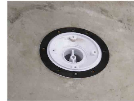
2. 泳池功能件预埋 Installation of embedded parts
